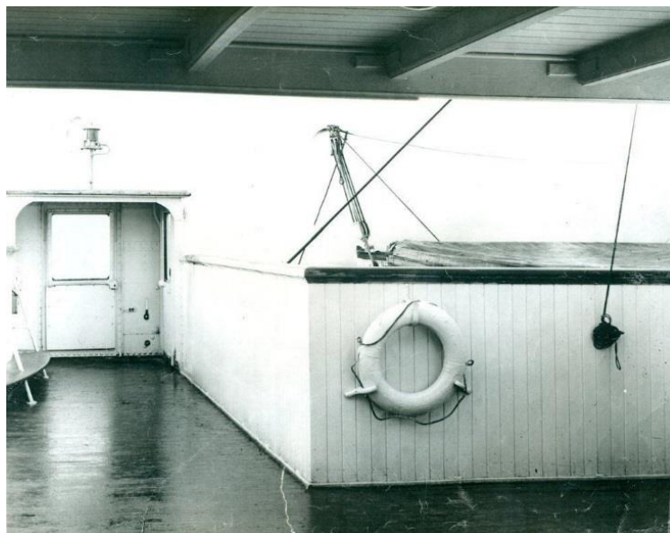
Navigating bridge roof Interior
