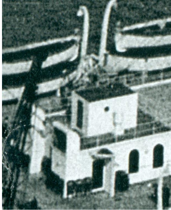
Elevator machinery room roof
