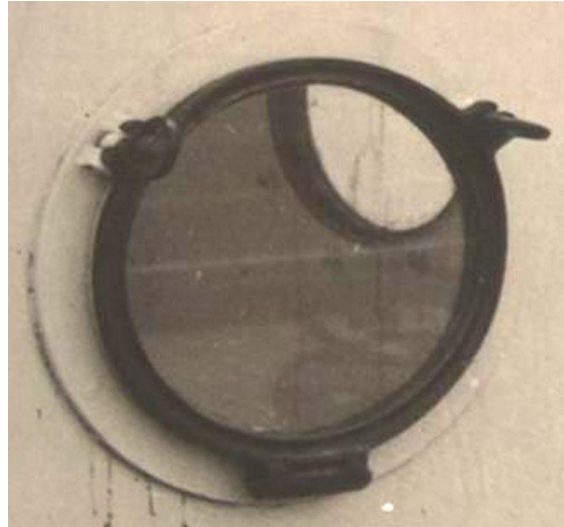
Hinged porthole on aft staircase weather cover
