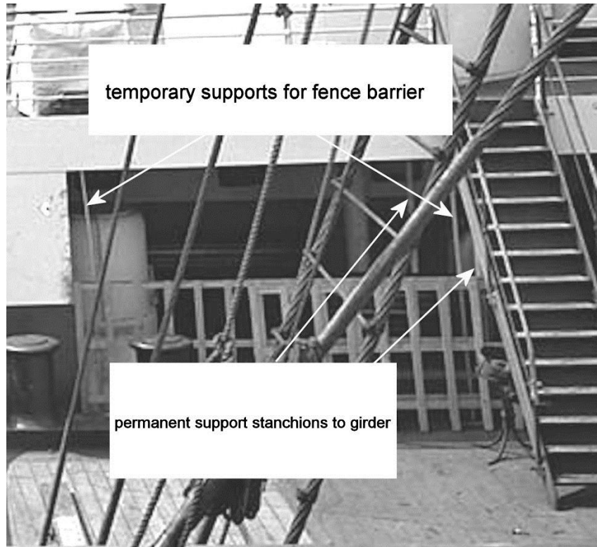
Permanent support stanchions to poop deck girder
